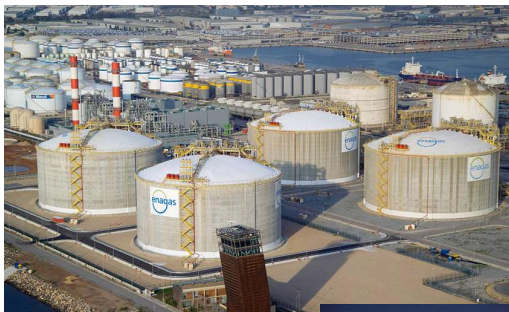
Power to Gas
